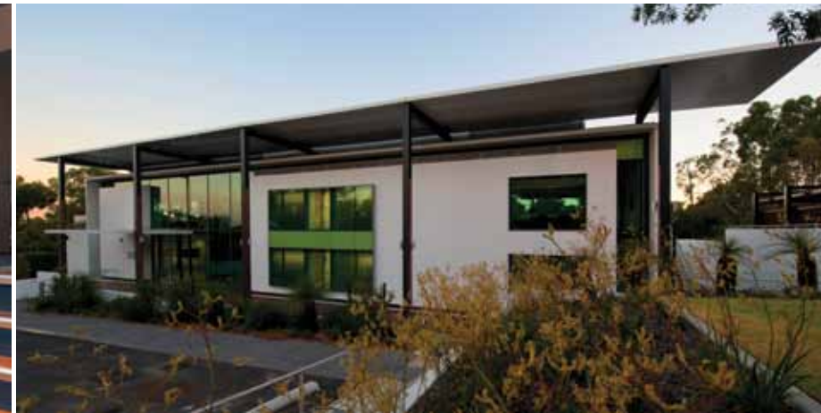
(Clockwise from left) The Centre's internal spaces are open and inviting, with extensive glazing affording views of the leafy campus. The concrete panels are crisply detailed with pencil round edges. The panels were designed and installed using accessible stainless steel bolts to allow ready disassembly. The thermal mass of the panels make a substantial contribution to the building's energy efficiency.
